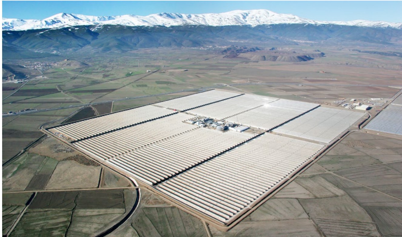
Photo ACS Cobra – Andasol 1-2
